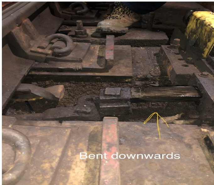
Photo 2 – Shows bent rod from track bed
