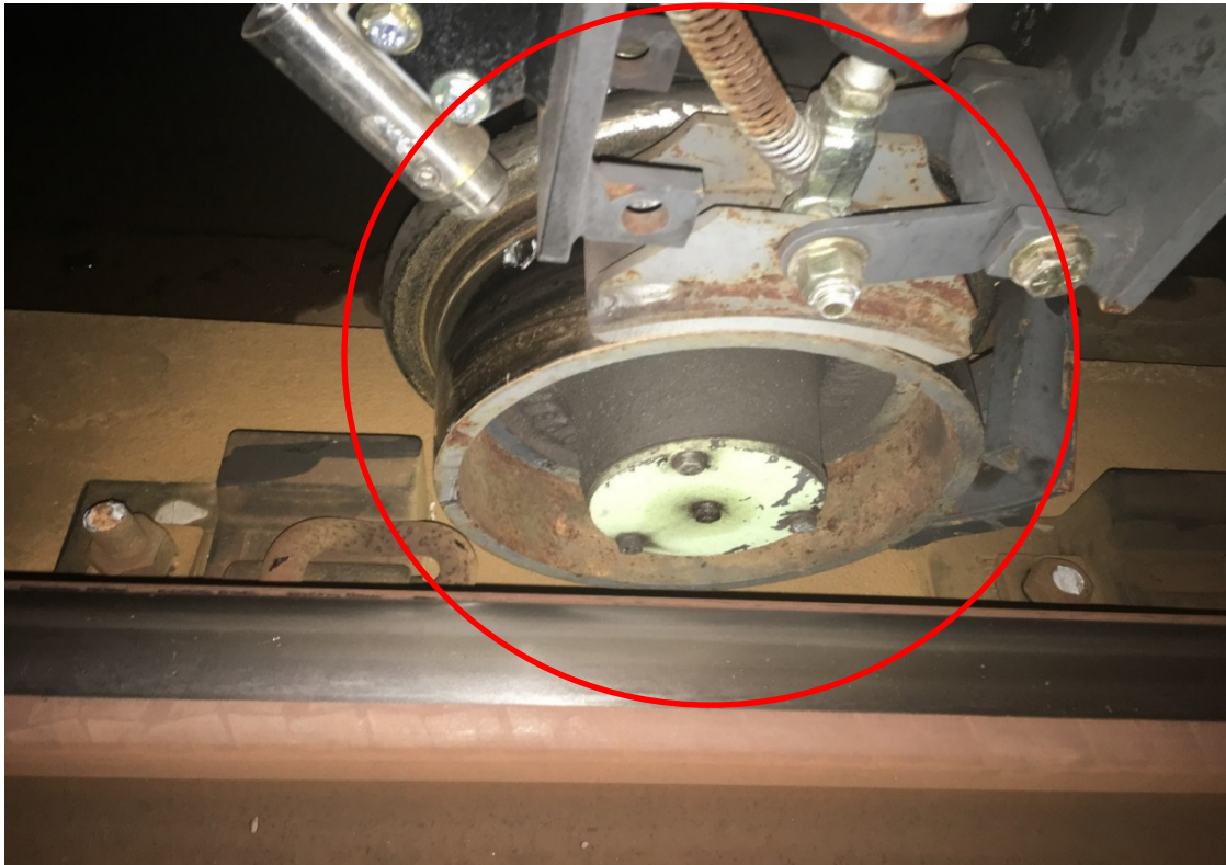
Photo 2 - Right Front Truck Derailed Gauge Side
