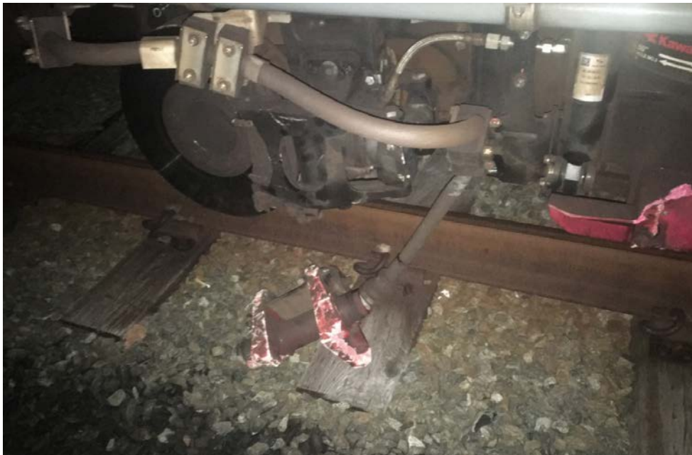
Photo 4 – Damaged Collector Shoe Assembly
