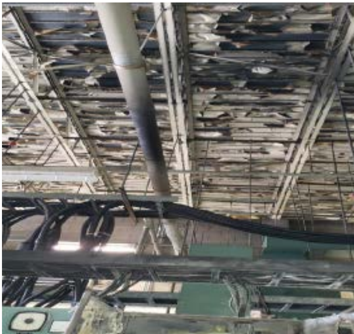
Picture 7 - C99 Transformer 2 Feeder Cable Conduit
