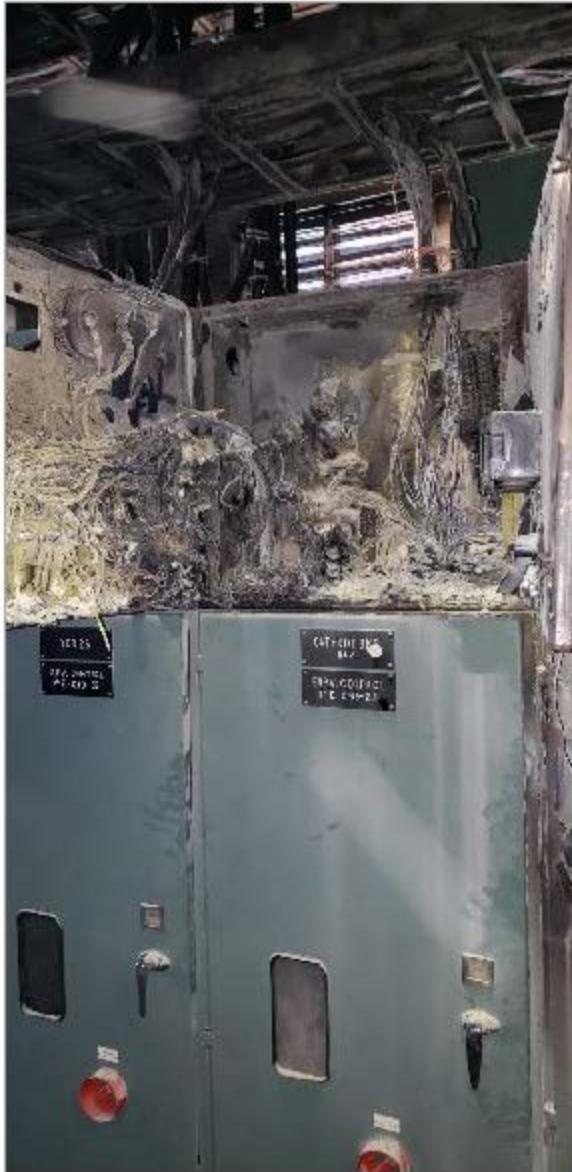
Picture 4 - C99 DC Breaker 22 Switchgear Cable Compartment and Breaker
