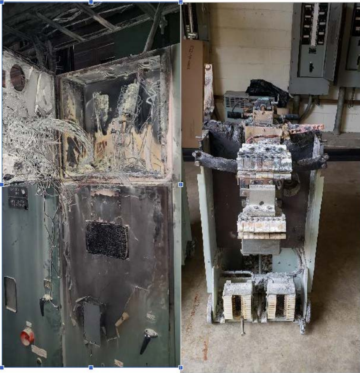
Picture 3 - C99 DC Breaker 50 Switchgear Cable Compartment and Breaker
