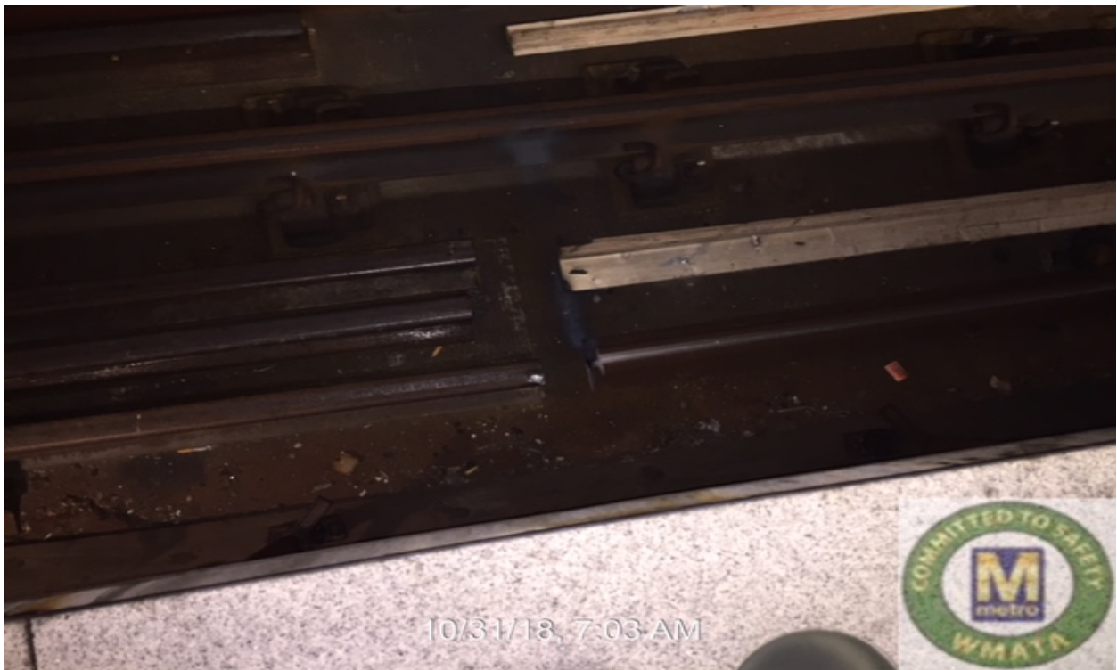
Photo 2 – Old rail was cut and moved
