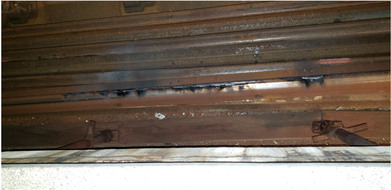
Photo 1 – Old rail that made contact with the collector shoe
