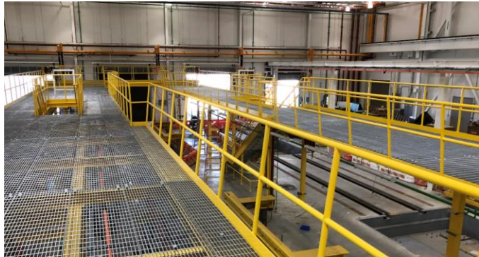
Photo 4 – Scaffolding is needed to reach railcar roof mounted equipment
