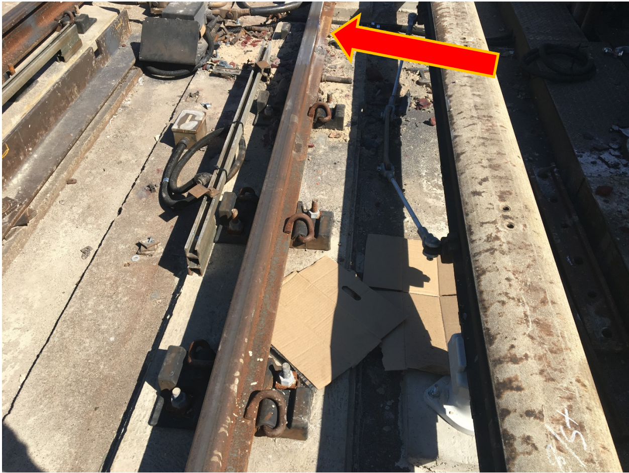
Photo 2 - Arrow indicates weld location
