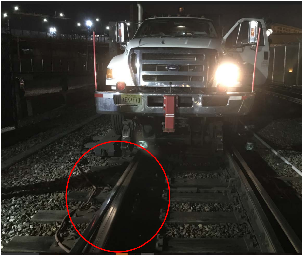
Photo 2 – Rail tucked on the left side of the rail indicating straight through move (Normal Position) for movement on adjacent track.
