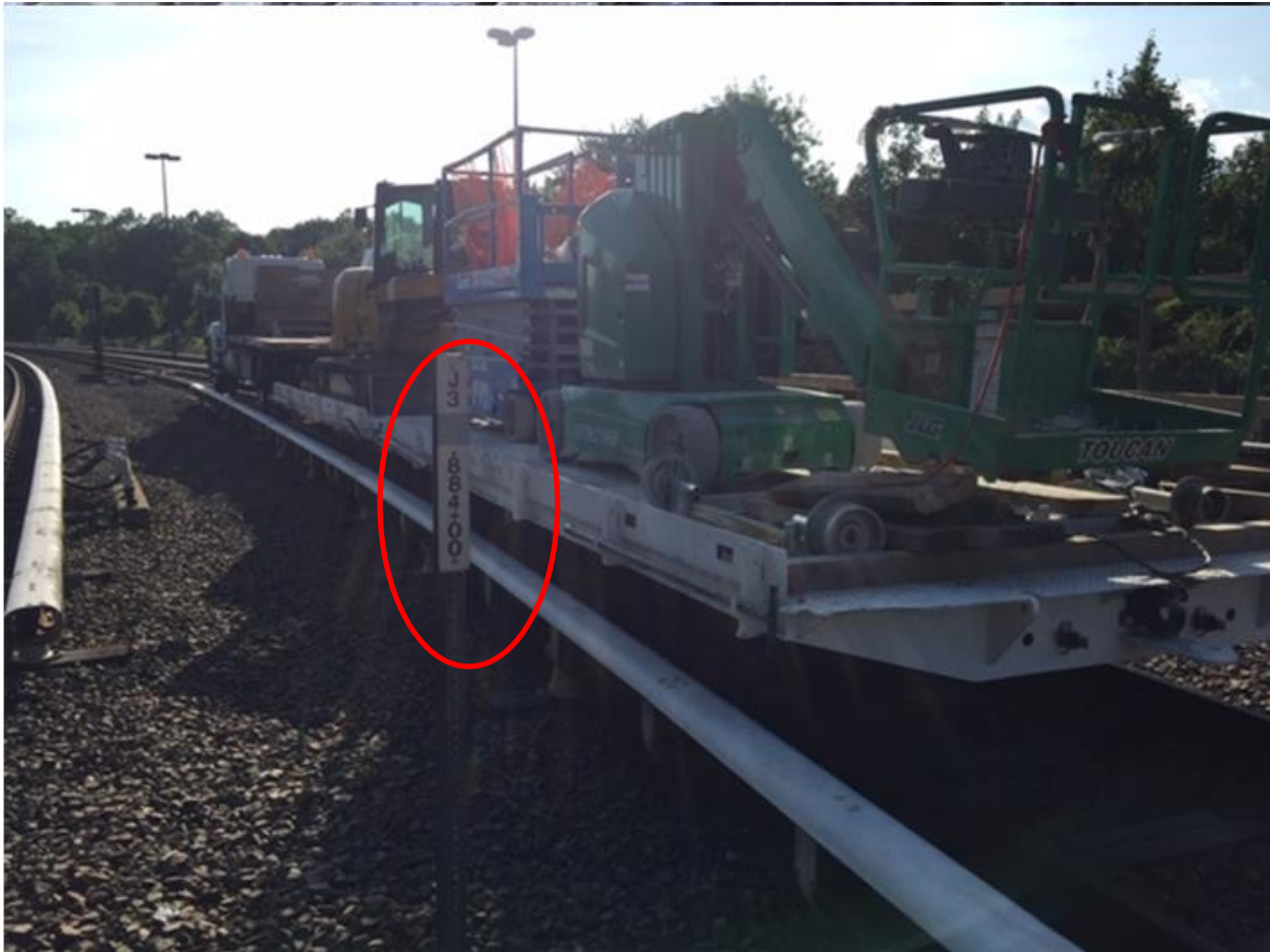
Photo 3 – CM location, Unit #801 Derailment, the weight distribution of equipment on the flat car
