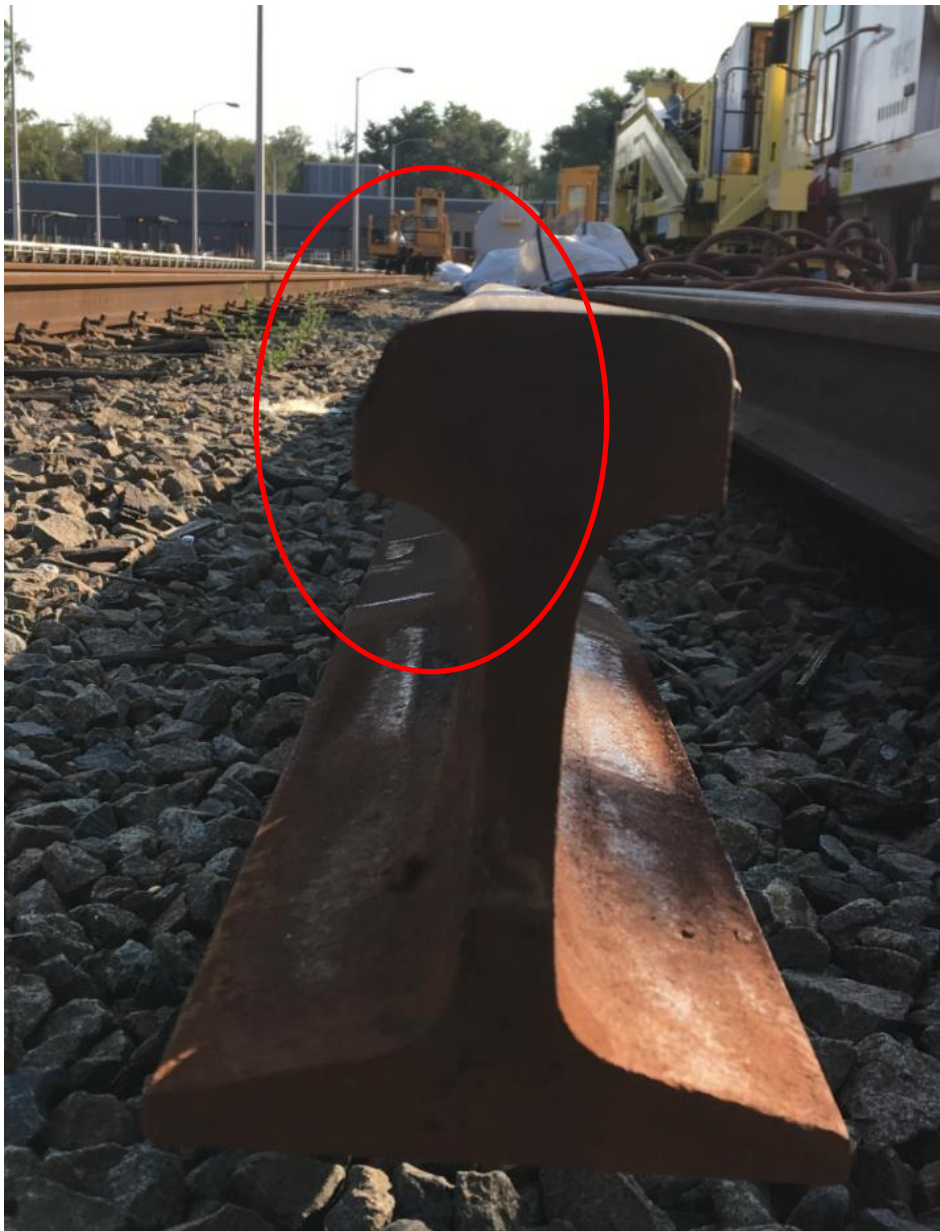
Photo 8 – Significant side wear of the rail
