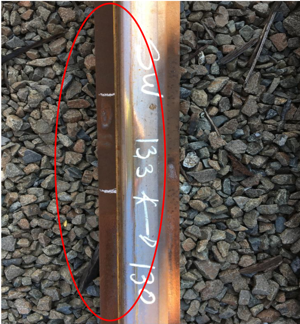
Photo 7 – Significant side wear of the rail
