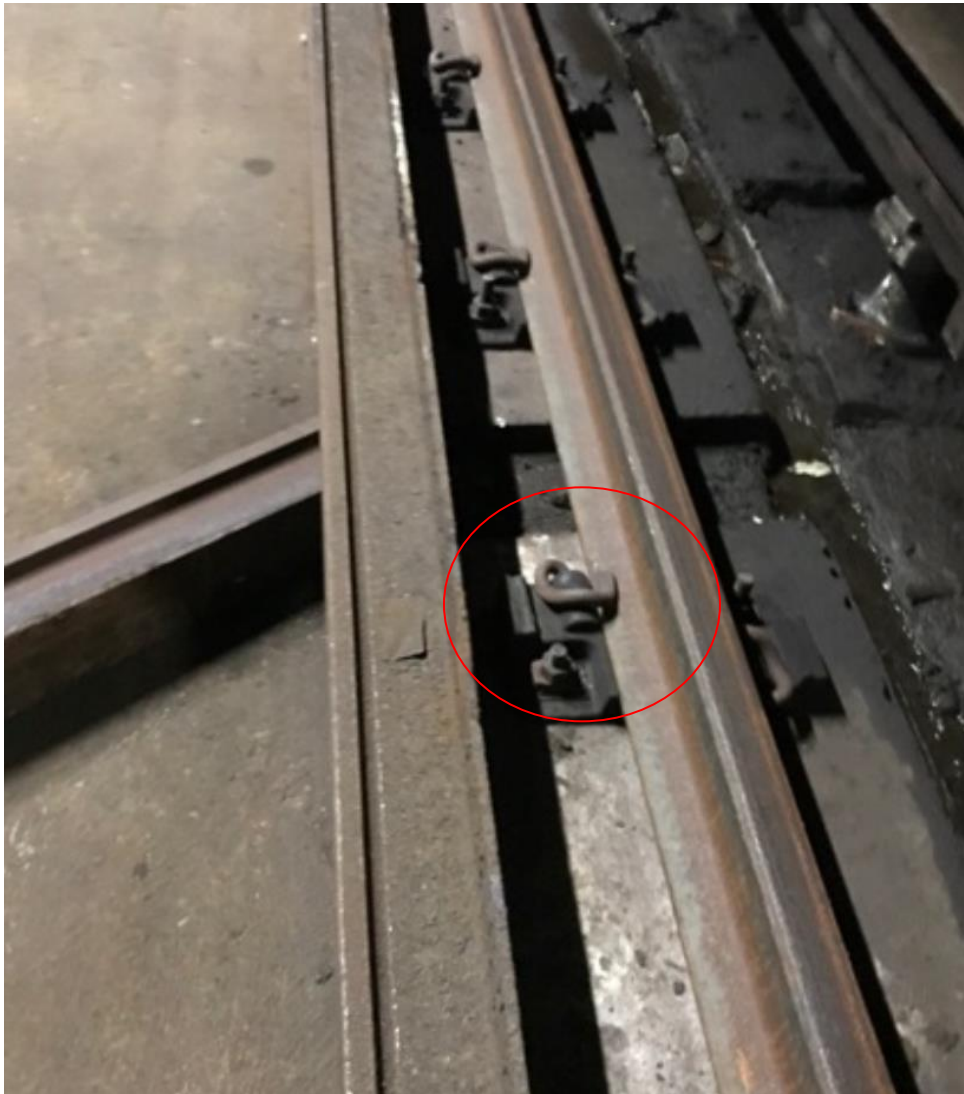
Photo 2 – Clips and fasteners installed on the New Rail
