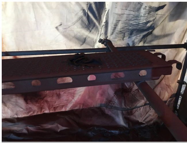
Photo 3 – Scaffolding platform area.
