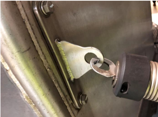
Photo 4 – The original inter-car barriers are showing signs of excessive wear at the connection link
