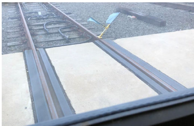
Photo 2 – Yard debris near the shop apron
