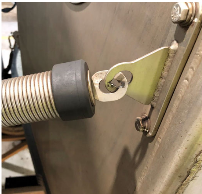
Photo 4 – The original inter-car barriers are showing signs of excessive wear at the connection link
