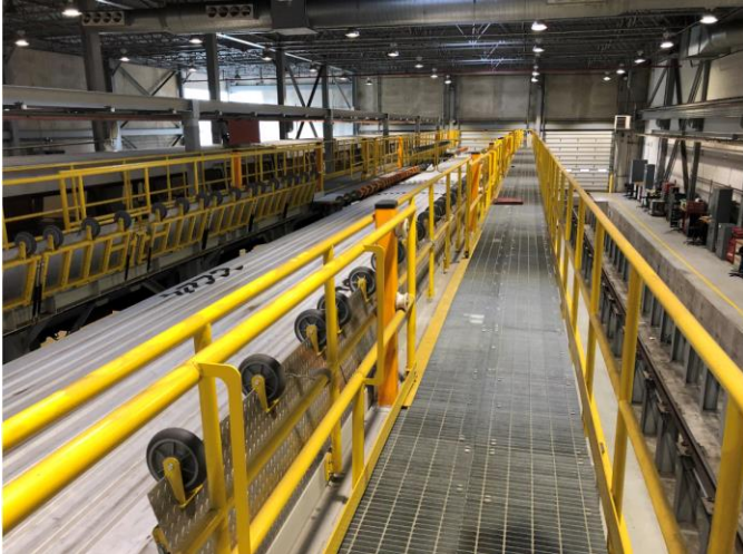
Photo 1 – New compact fixed scaffolding structure to reach railcars roof mounted equipment
