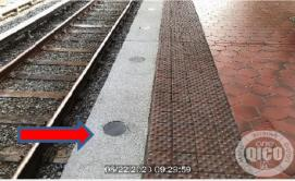
Multiple edge warning ADA (bumpy tiles) missing/broken Track 1 North End
