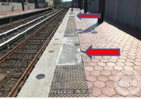
Multiple public address system speakers missing (Platform canopy Track 1 and Track 2) Remedial Action Required? No
