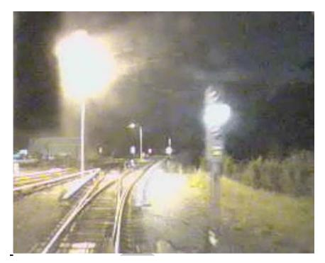
As the Train Operator approached, E99-160 was displaying a red signal aspect; the Train Operator proceeded to pass the signal.
