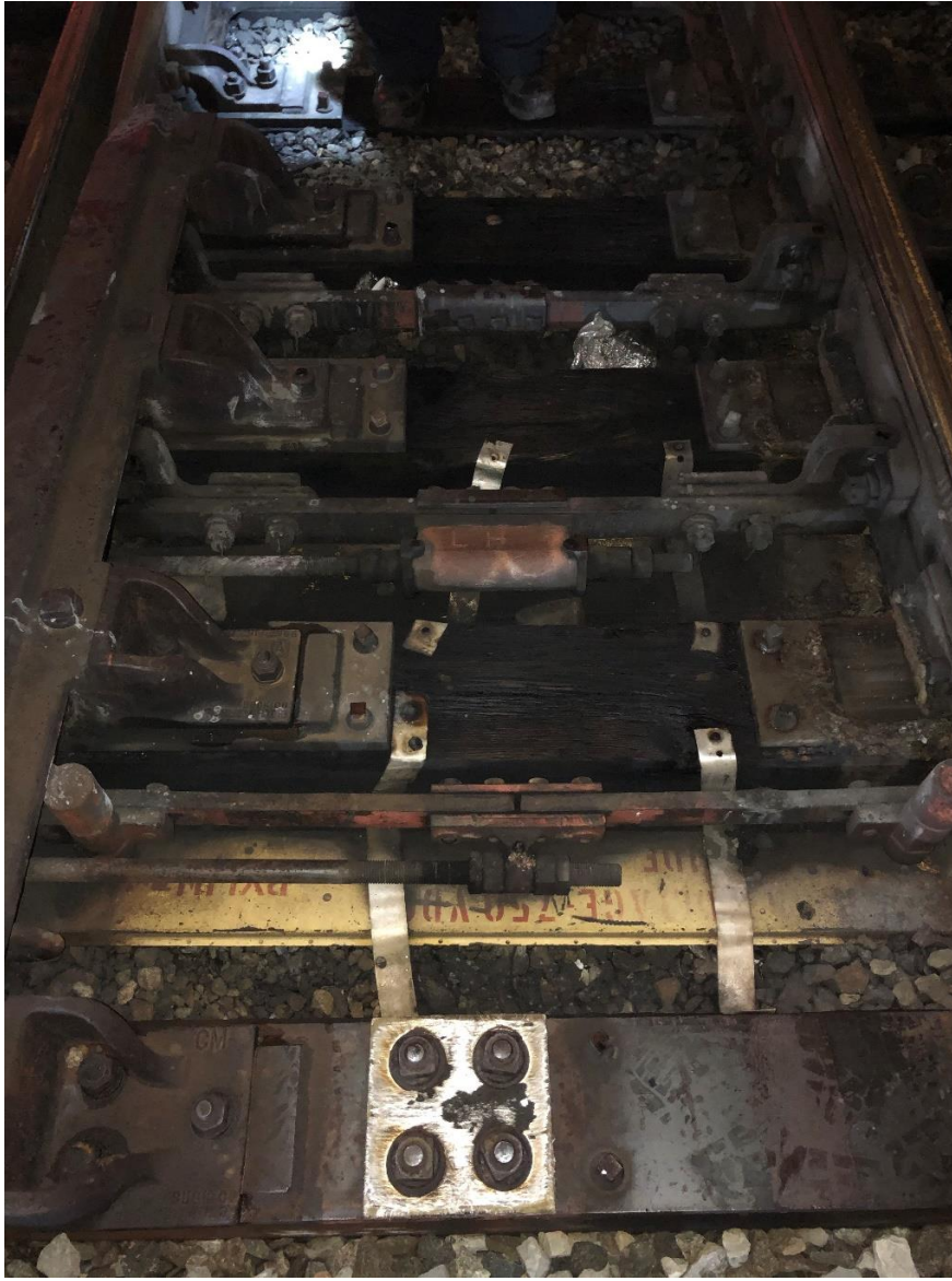
Photo 2: ATCM Photo – Switch 141B with switch cover removed and showing no signs of damage.
