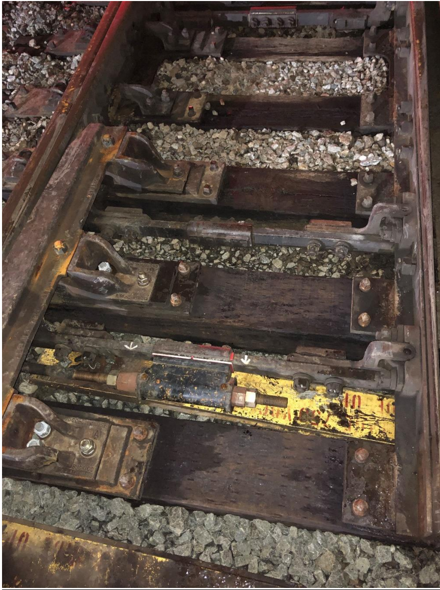
Photo 3: ATCM Photo – Switch 143 with switch cover removed, showing no signs of damage.
