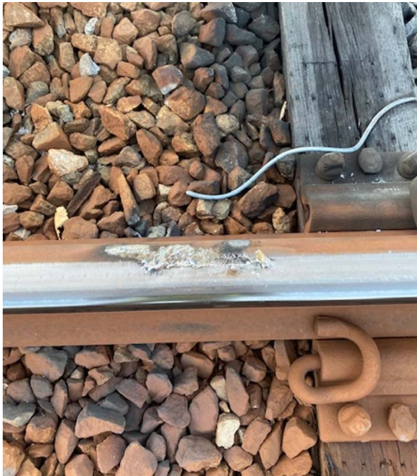
Figure 11: Observed burn marks on the running rail near the pull-apart location.
