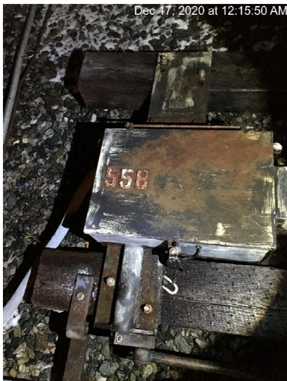
Photos #6 and #7: Incident train traveled through Switch 55B (clamped) after passing Signal D99-54 (Red). ATC found no damage.
