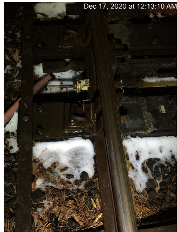
Photos #4 and #5: Incident train traveled through Switch 57B (clamped) after passing Signal D99-54 (Red). ATC found no damage.
