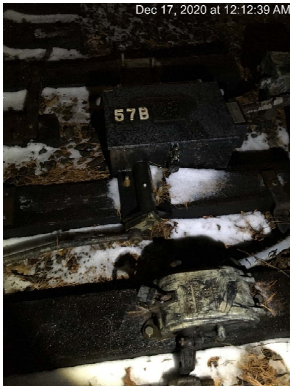
Photos #4 and #5: Incident train traveled through Switch 57B (clamped) after passing Signal D99-54 (Red). ATC found no damage.
