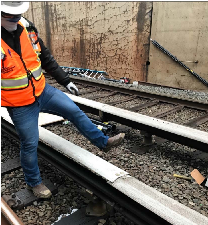
Figure 2 – The Injured Contractor stepped over the third rail leading with their left leg.
