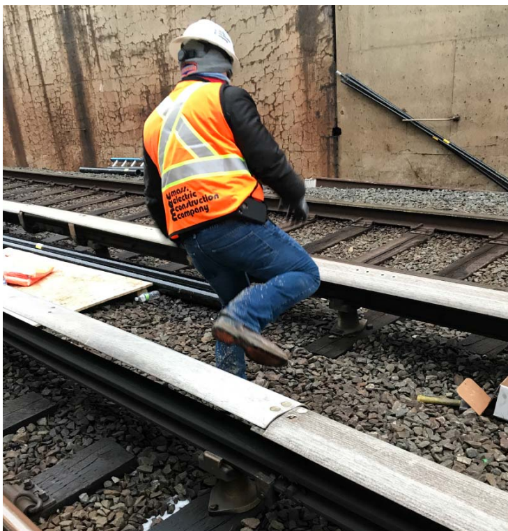
Figure 4 – The Injured Contractor then stepped over the third rail and pivoted on their planted left leg, and subsequently fell between both of the third rails.
