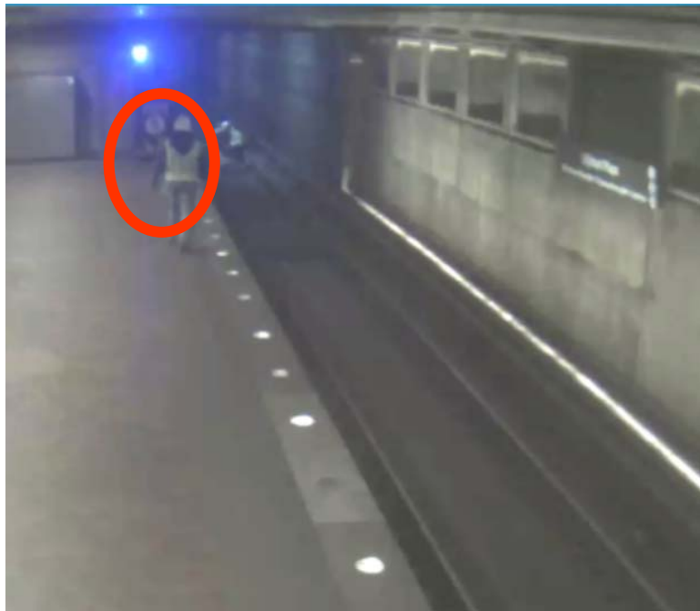
Figure 4 - Based on the CCTV, at 02:35 hours, the RWIC and three contractors entered the roadway to engage in work activities without being RWP trained and qualified. Additionally, the PLNT Craft Supervisor arrived on the scene and walked beyond the station's end-gate while the three contractors were retrieving debris from the roadway.
