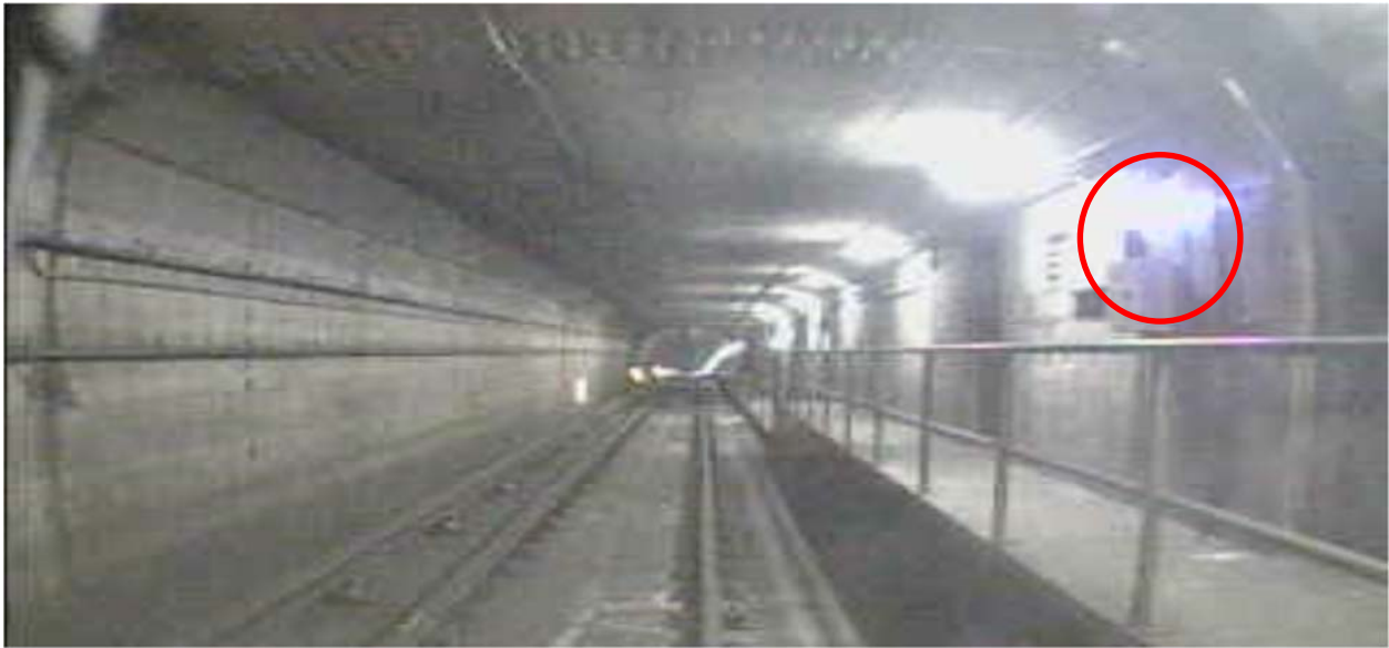
Train ID 907 Train Operator begins to move. Use the blue ETS station to the right as a marker. ETS boxes are located every 800 feet.
