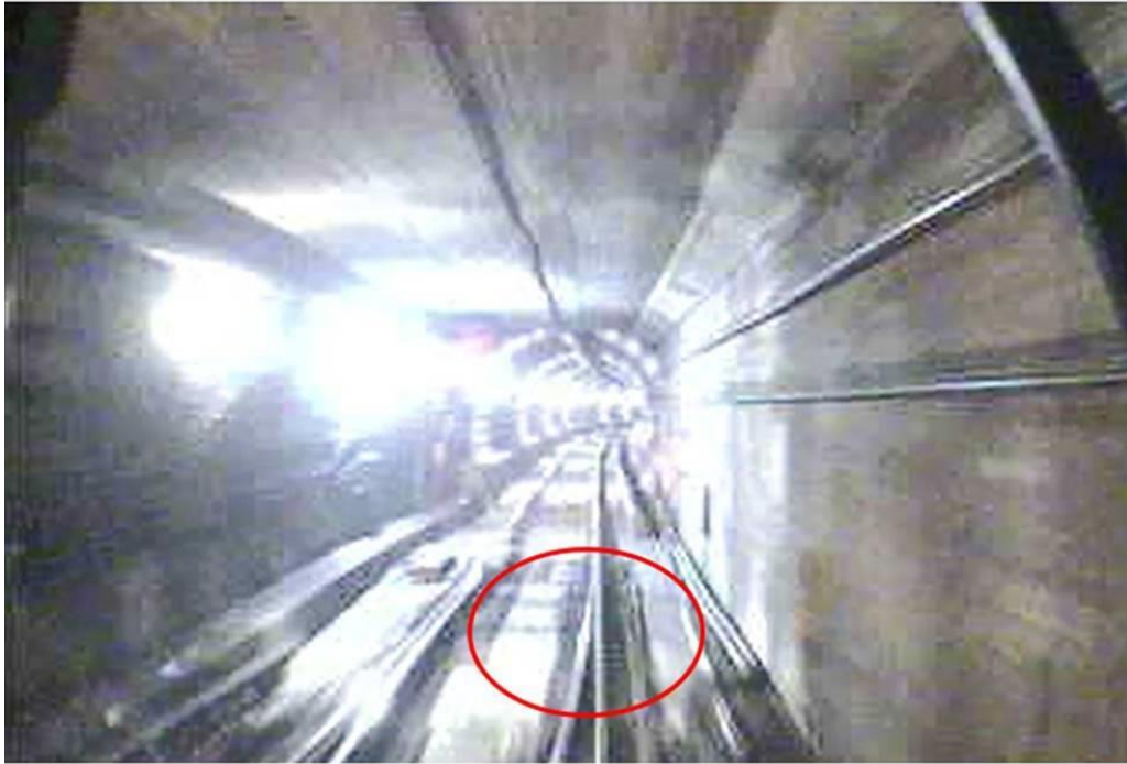
Photo 3 – E03 Switch 3B in the reverse position.
