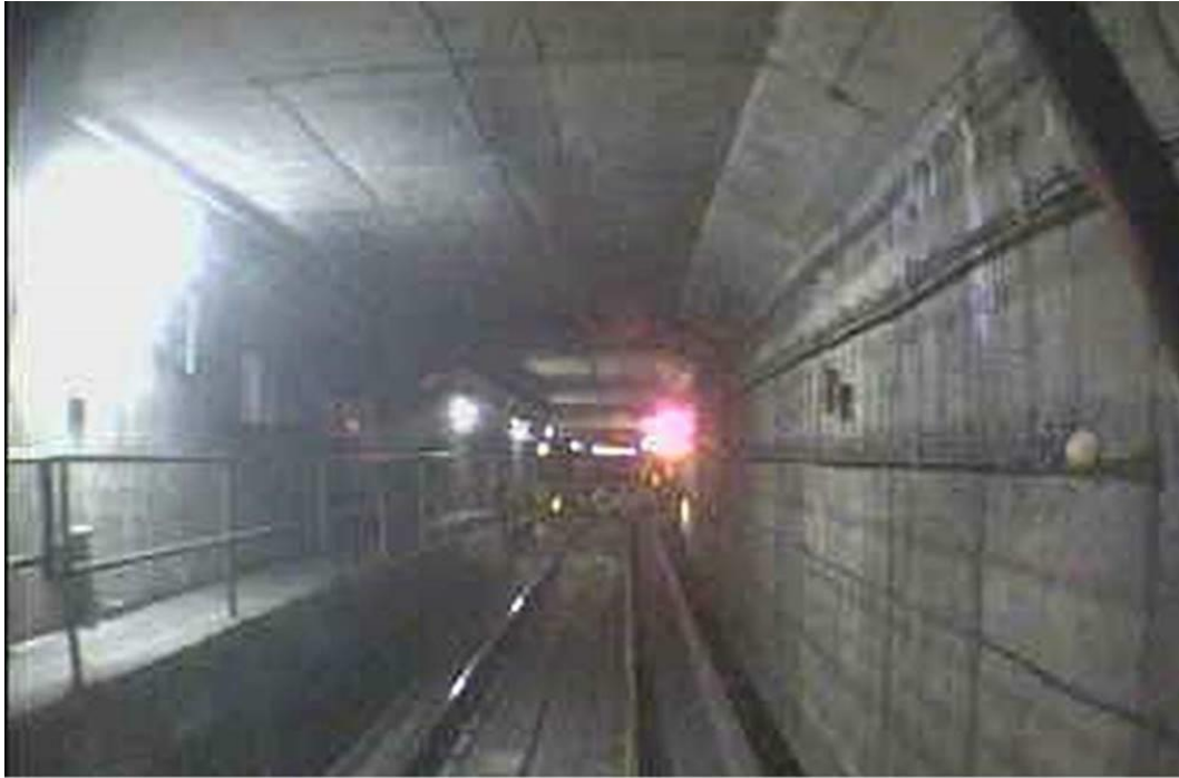
Photo 1 – E03-08 signal displaying a red aspect as seen from the 8-car marker.
