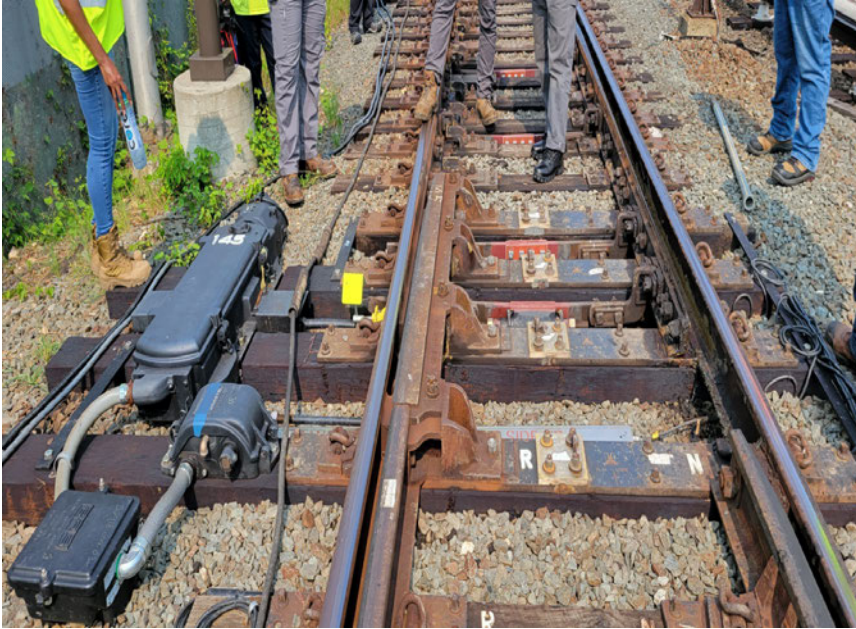
Switch 145 showing cable interference
