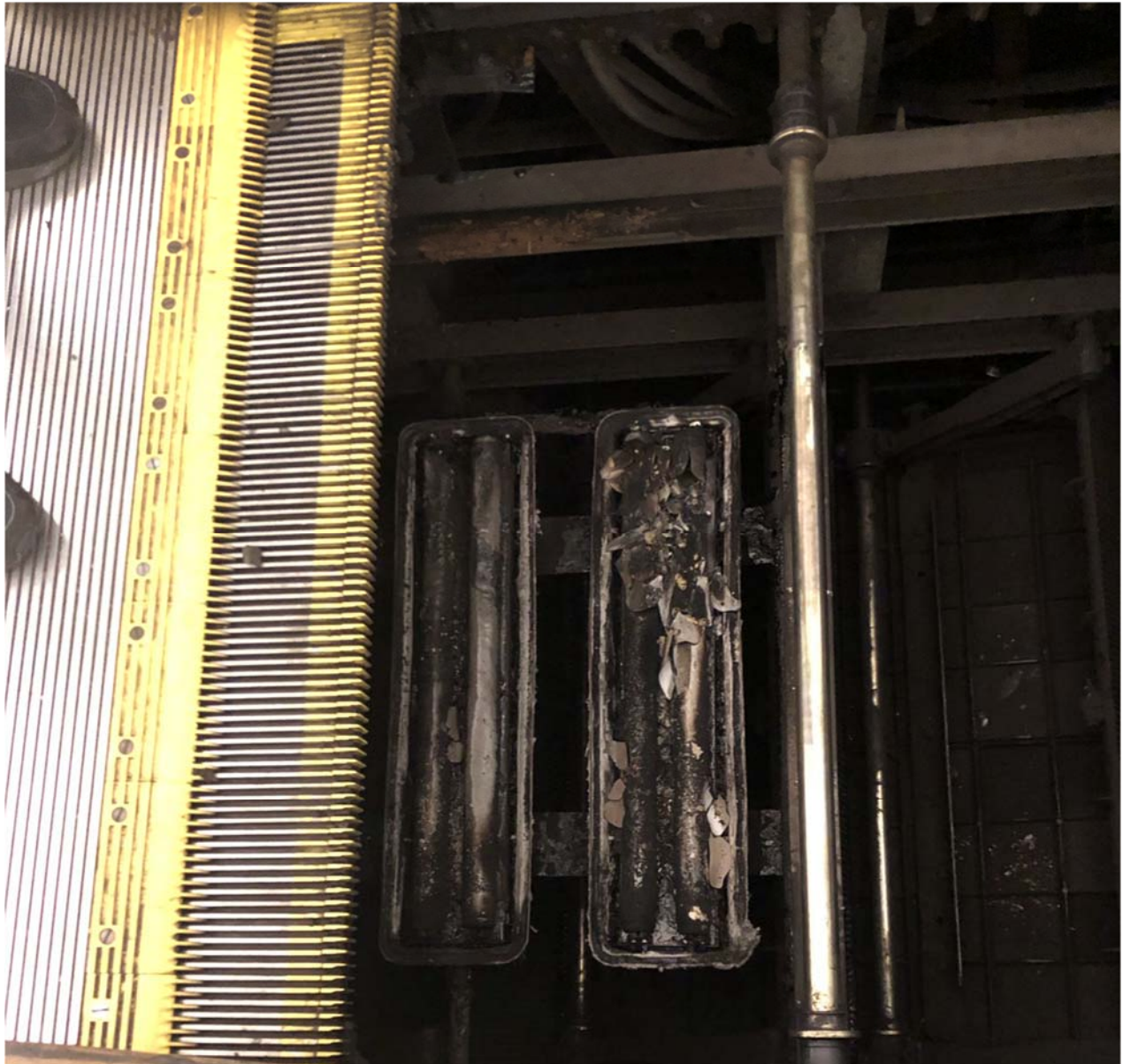
Figure 6 - Florescent Bulbs Inside Lower Portion of Escalator #4
