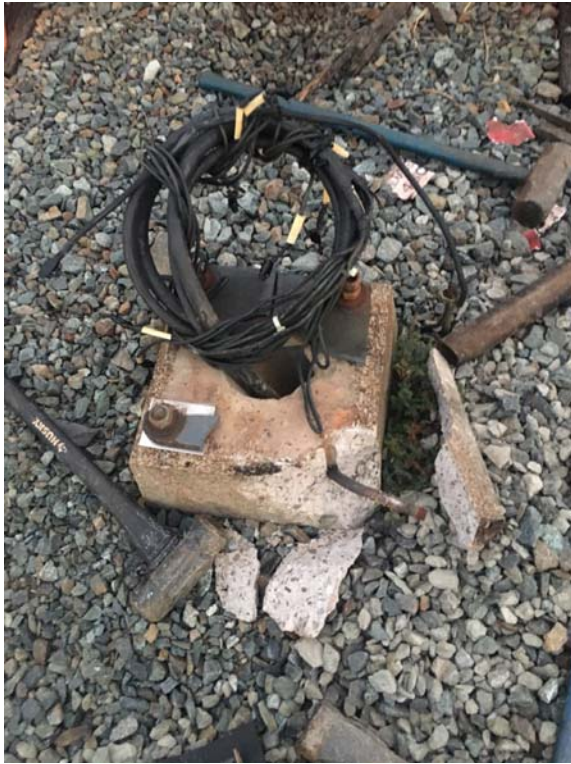
Figure 2: This image shows the base of A99-146 signal, which will need to be completely replaced.
