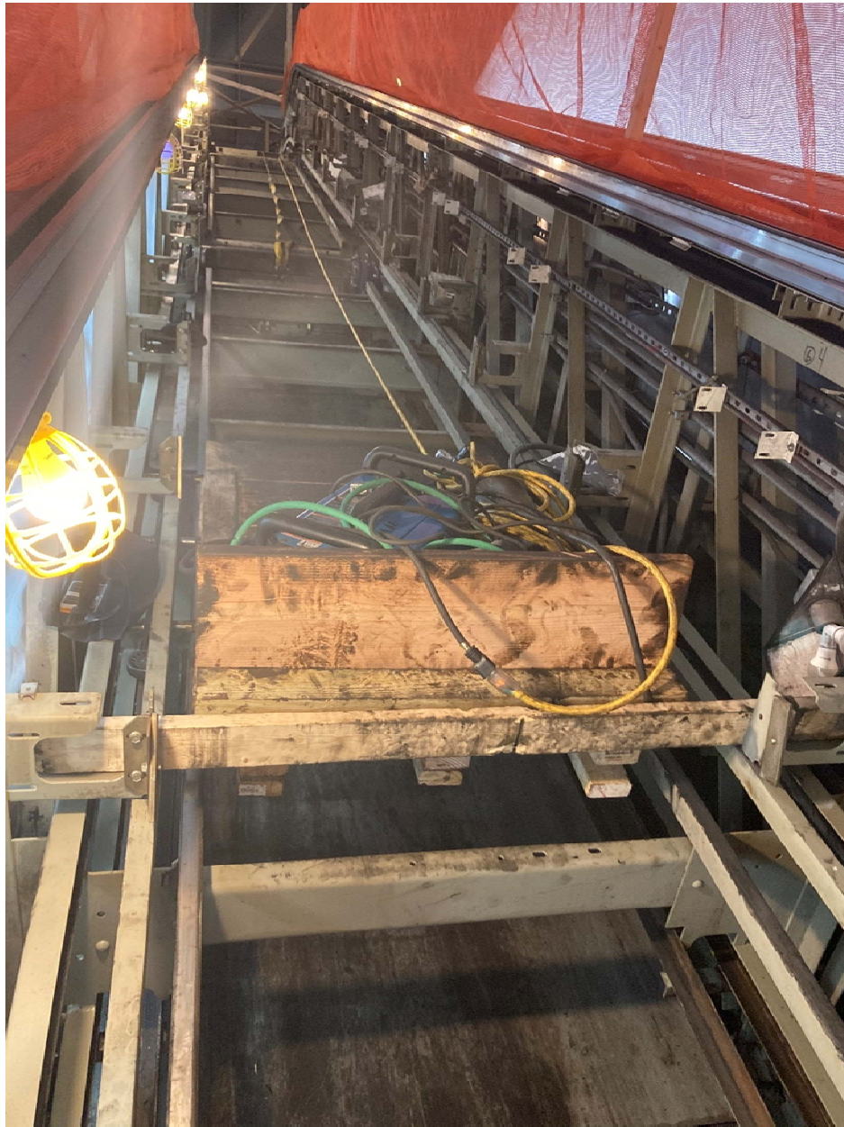
Photograph 3 – Bottom view of work sled in escalator truss.
