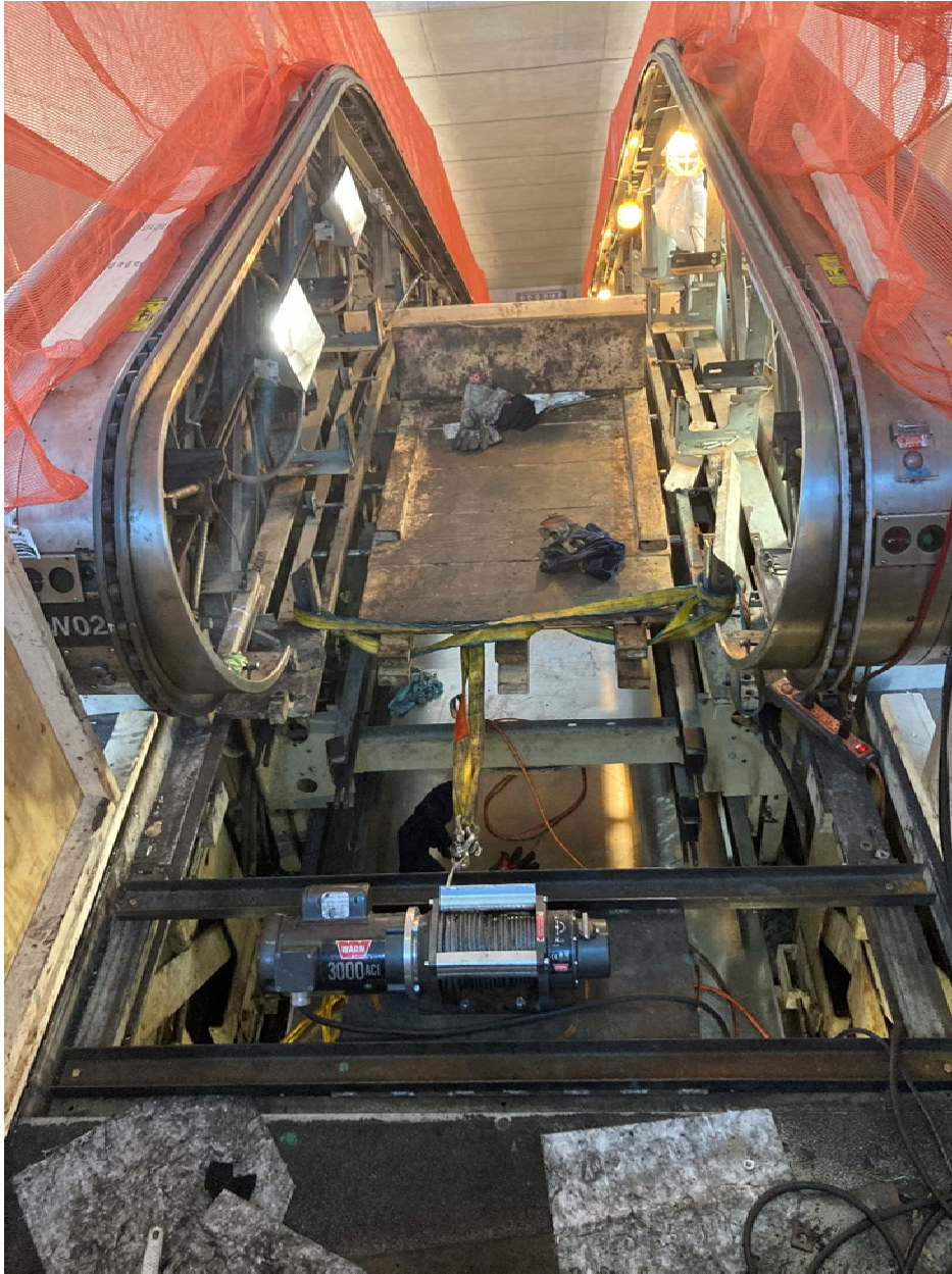
Photograph 1 – Top view of Escalator W02 displaying the winch and work sled setup.
