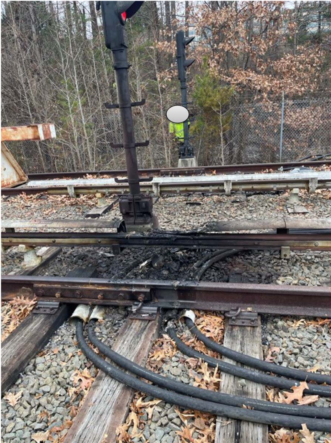
Figure 6 – Additional angle of incident location showing damage to ATC cables, third rail, cross ties, insulated joint bar and cover boards.
