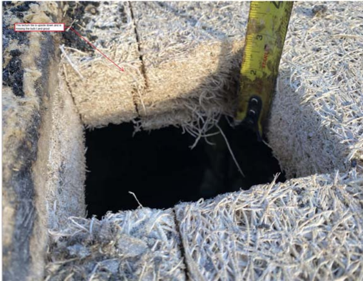
Figure 15: Cutting of tectum from the roof of T-36.
