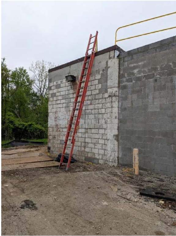
Figure 3: Egress ladder on to the roof, with proper three-foot overlap, located on the North-West Corner of T-36.
