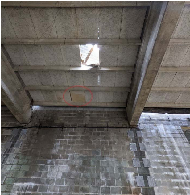
Figure 11: Water-damaged tile within the vicinity of the incident site.
