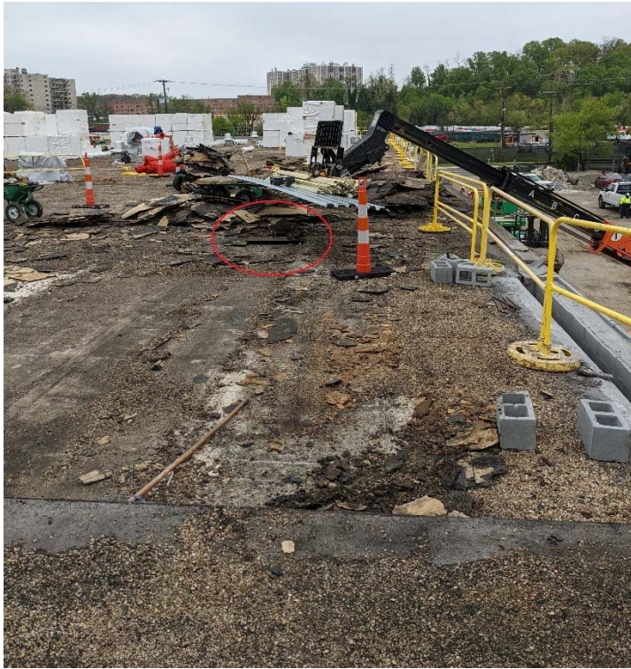
Figure 6: Northwest Corner orientated to the South, missing tile creating the hole can be observed from the safe area. Forklift can be observed to the right of the hole.
