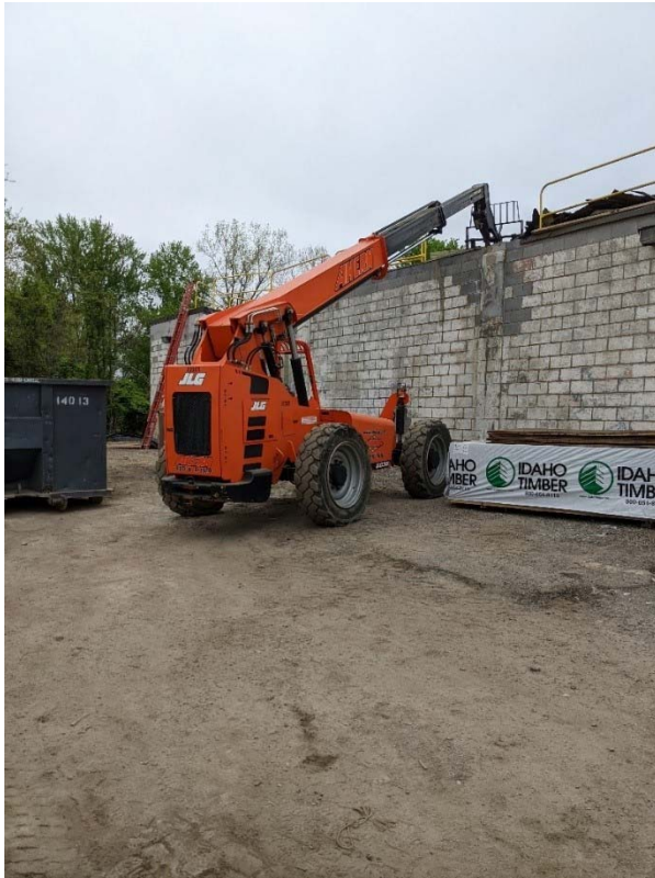
Figure 5: Forklift stationed on the ground with fork overhanging the roof to provide supplies.
