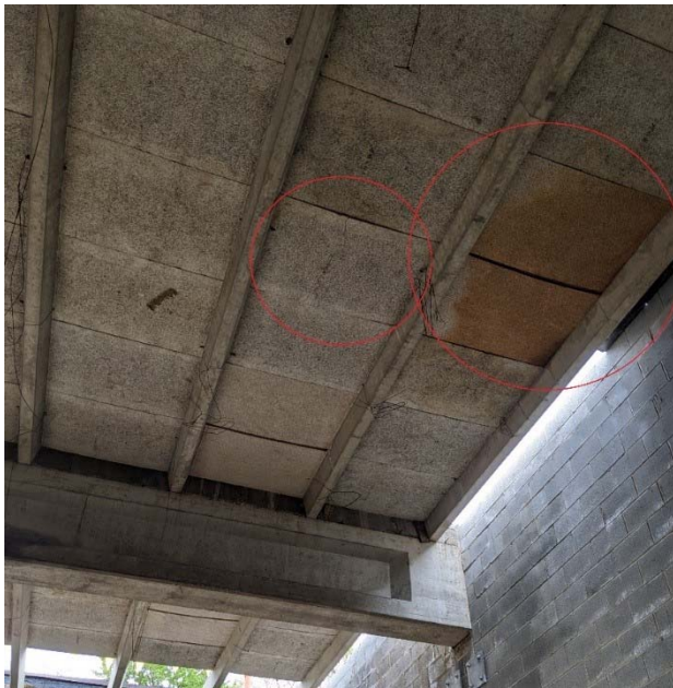
Figure 12: Two water-damaged tiles and a structurally compromised tile near the East wall.
