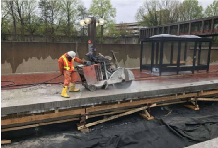
Figure 7: Granite being cut by an ACC employee with an industrial saw.
