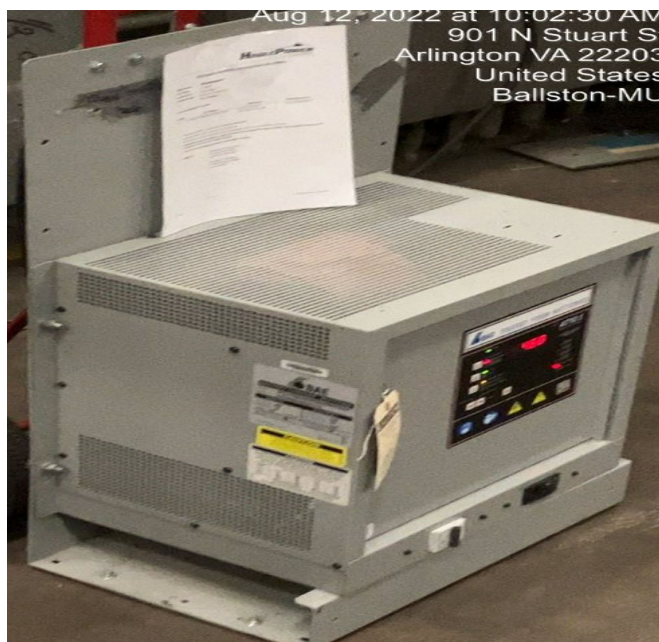
Figure 7 - Temporary Charger installed for mitigation purposes (photo taken prior to installation).
