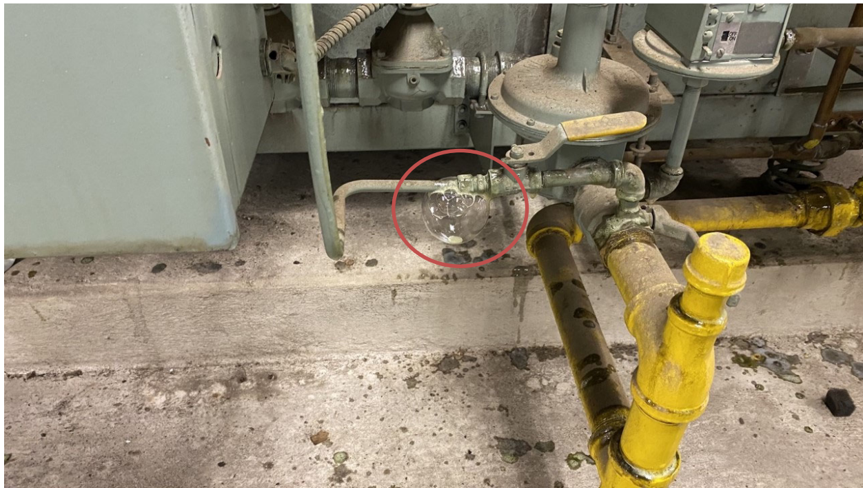
Figure 2 - Gas leak located on HVU#1 using bubble test method.
