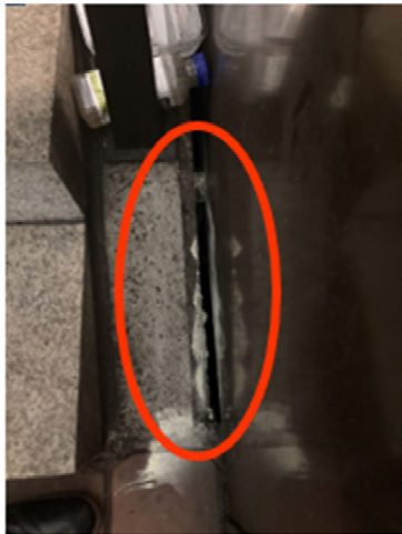
Image 1 - Gap between escalator six and the staircase.
