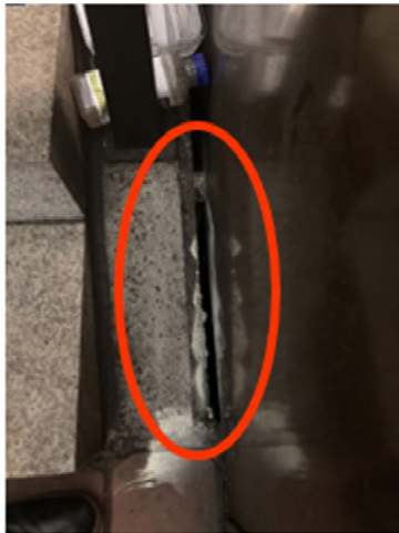
Image 1 - Gap between escalator six and the staircase.
