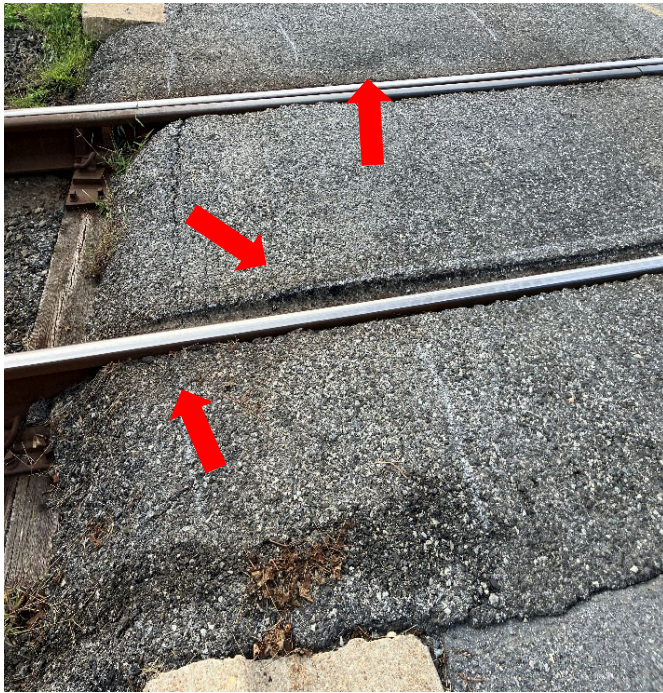
Figure 6: Shows the asphalt at the beginning of the grade crossing that is uneven, with some ridges and bulging.
