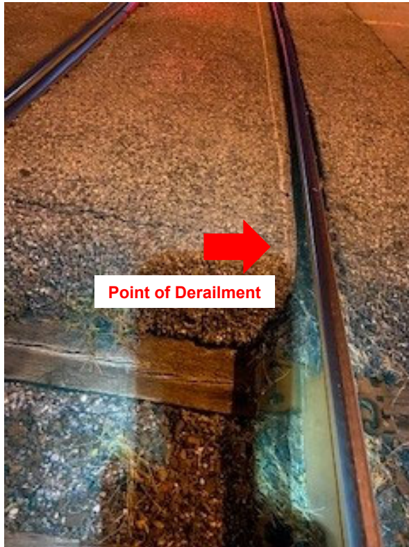
Figure 3: Shows the view looking at the beginning of the grade crossing where the point of derailment occurred.
