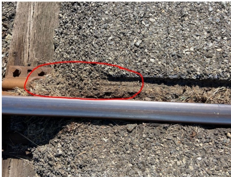
Figure 8: This image shows debris that was observed in the flangeway.
