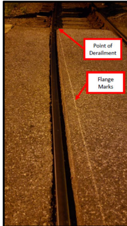
Figure 2 – Point of derailment/Flange Marks
