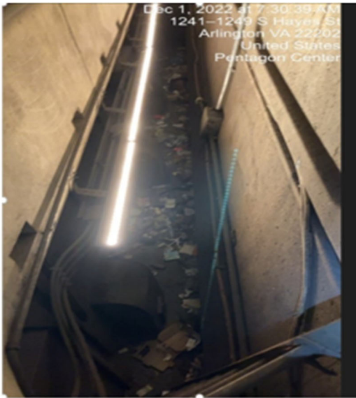
Image 1 – Burned trash and debris located behind the parapet wall.
