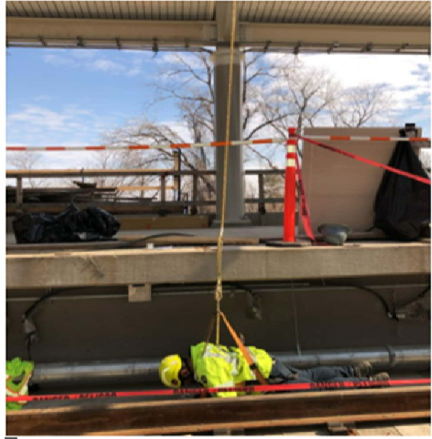
Image 1 & 2 – Photo of the top of the canopy depicting the open bay and photo of the end state of the fall arrest system demonstrated by WMATA SAFE personnel.
