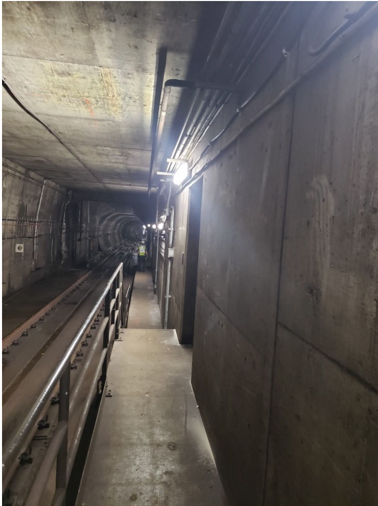
Figure 3 - New Lighting Installation at Medical Center Track 1
