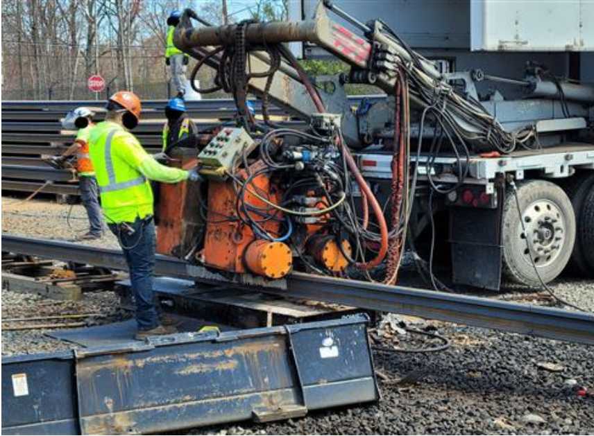
Inspection Orange Line Rail replacement staging 4.jpg
