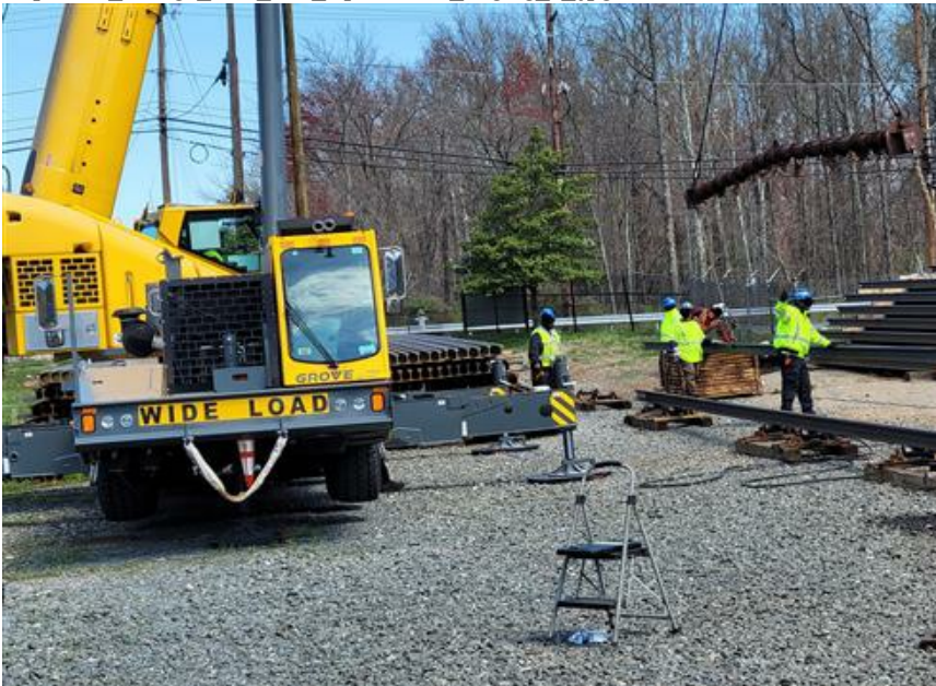
Inspection Orange Line Rail replacement staging 3.jpg
