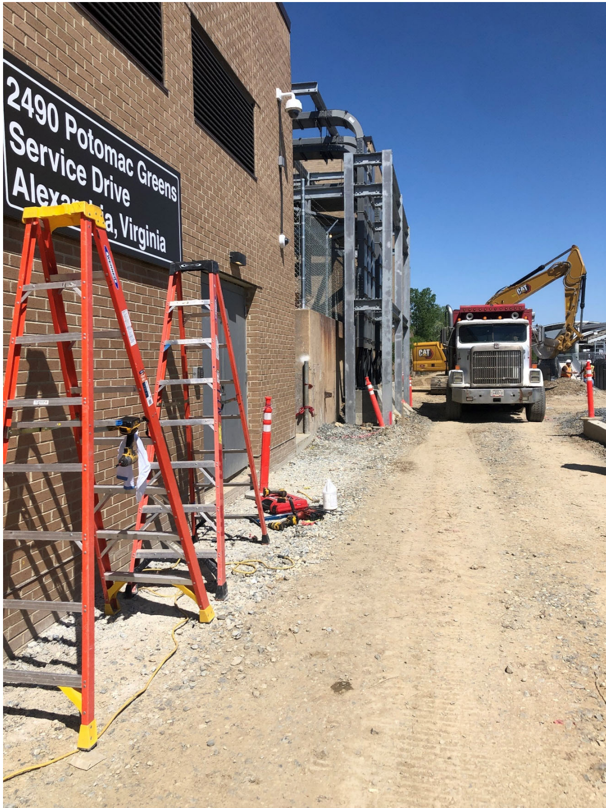
Image 2 – View of the Gelberg Signs Employee’s work location setup within the construction zone at the Potomac Yard Station. Note cords and uneven ground beneath the ladders’ footing.
