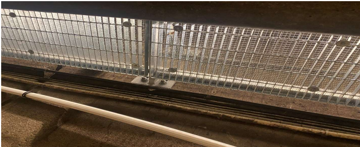
Figure 13 Metal Grates installed behind the Parapet walls located at Gallery Place Station
