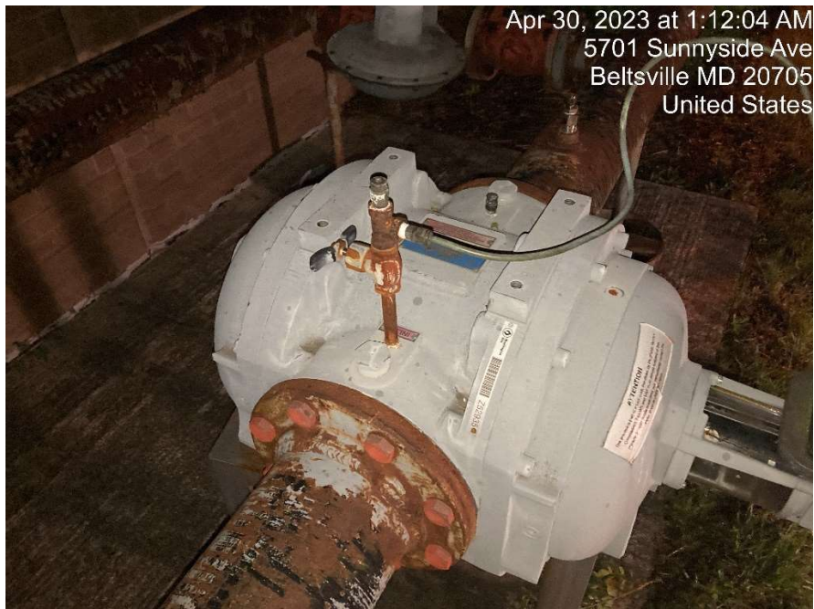
Image 3 - Top View of Leaking Gas Meter on Exterior of Building B (S&I Shop)
