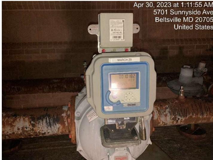
Image 1 - Front View of Leaking Gas Meter on Exterior of Building B (S&I Shop)
