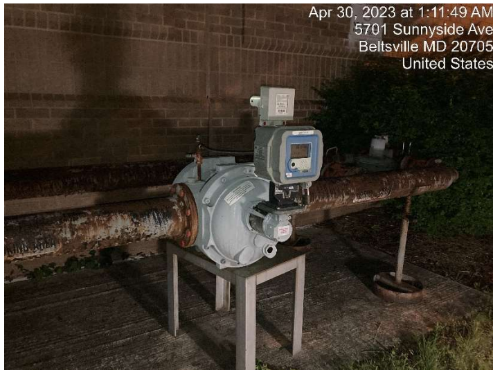
Image 2 - Side View of Leaking Gas Meter on Exterior of Building B (S&I Shop)
