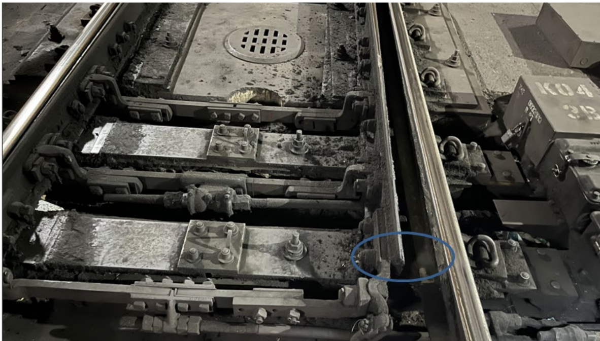
Image 2 – Image of damage at switch point 3B.
