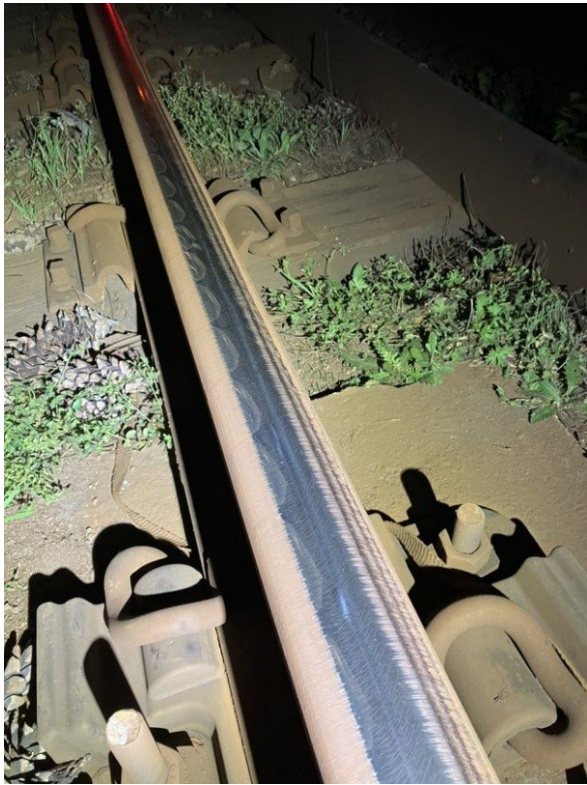
Figure 5: The rail markings switched to a swirling mark at approximately 20 feet prior to the point of derailment.
