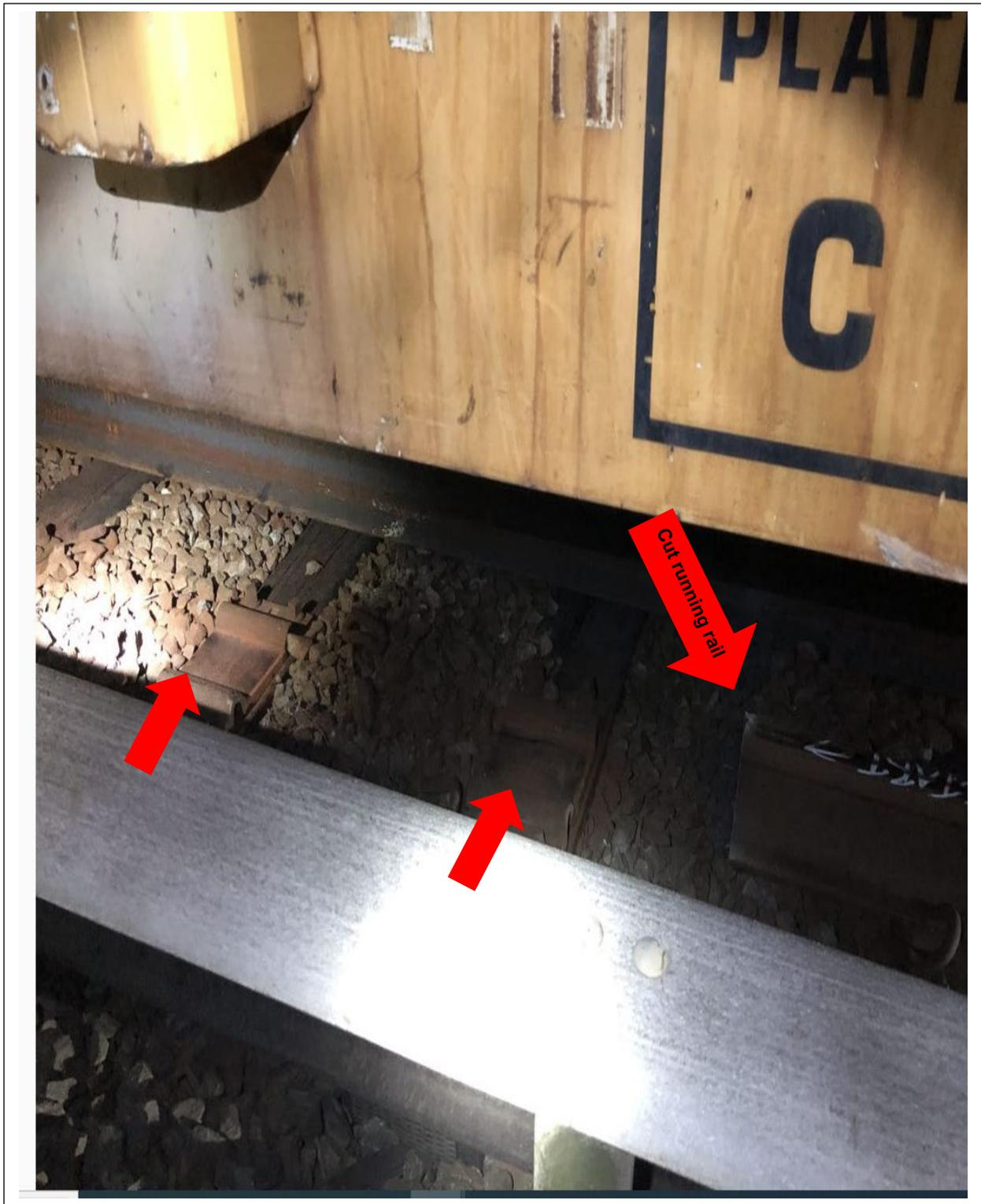
Figure 12 Cut running rail at the point of derailment.
