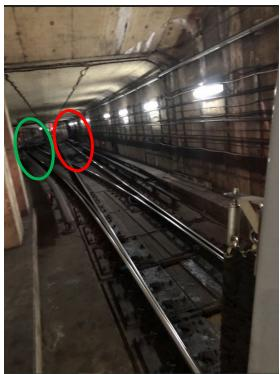
Figure 6: The green circle is where the Train Operator was supposed to go, and the red circle shows where the train was aligned for before it stopped.
