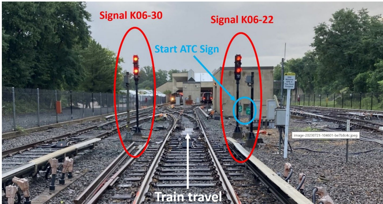
Photograph 1 – Yard Lead 2 with Signal K06-30 on the left and Signal K06-22 on the right. The Start ATC sign and “S” marker are pictured on the right side of Yard Lead 2, adjacent to Signal K06-22.
