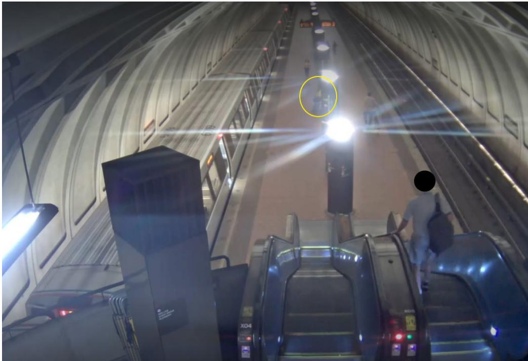
Image 2 – The TRST RWIC and TRST Track Inspector are observed at Medical Center Station seated, orientated towards track 2 at 09:34 hours.
