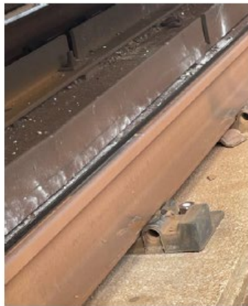
Figure 10: Debris around EGR
