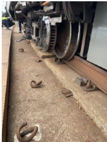
Figure 6: Derailed Left Wheel of Lead Axle
