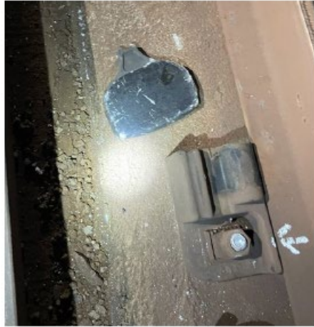
Figure 3: Sheared Field-Side Stud
