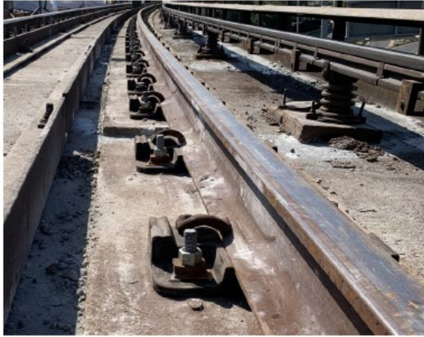
Figure 17: New SW-31 Installed
