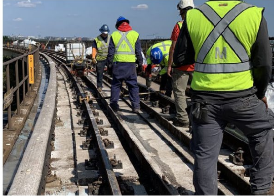
Figure 15: Track Gauge Verification
