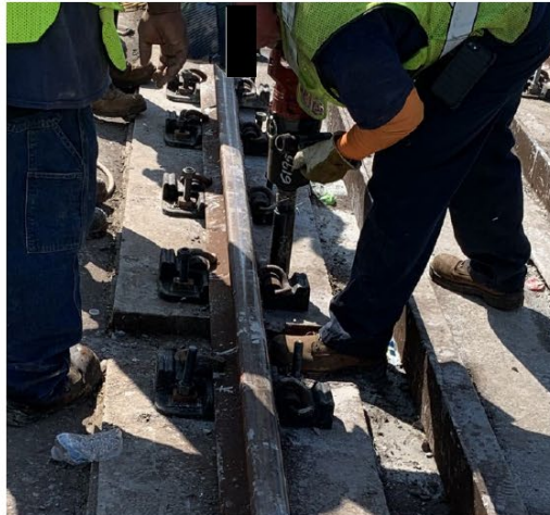
Figure 16: Fastener Torquing
