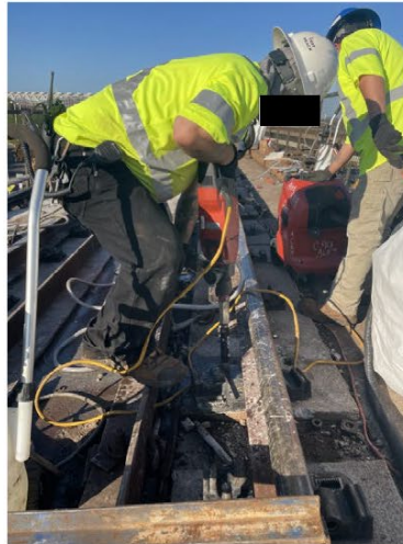
Figure 14: Core Drilling New Studs
