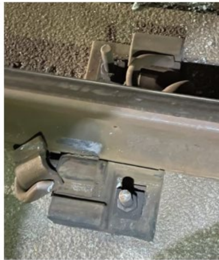
Figure 4: Damaged Fastener
