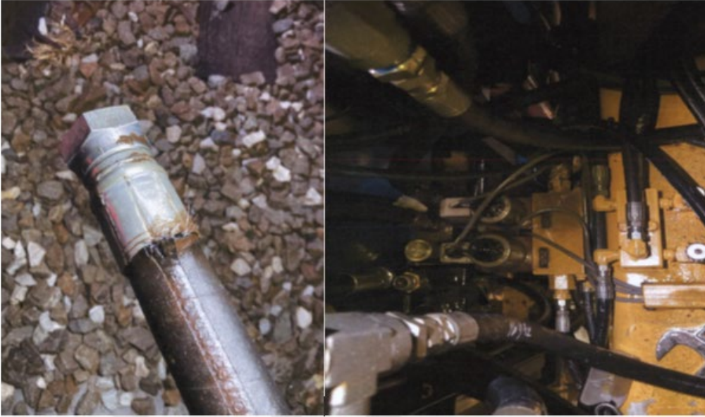
Figure 8 - Tamping Unit T004 broken hydraulic fluid line and the repaired hydraulic fluid line.
